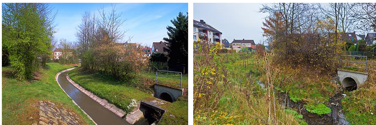
Fig. 4. Comparison between an unrestored (left) and a restored section (right) (Dortmund Aplerbeck) (Source: EmscherGenossenschaft).
